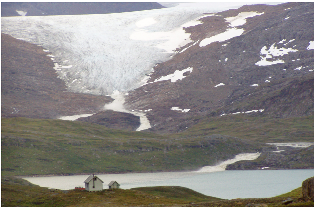
Figure 13-5 Water escaping from a 2.3 km long tunnel under the Rundvassbreen glacier. The photo is taken in the afternoon on Monday 29 August by Hans Martin Hjemaas, Elkem Energi Siso AS.
