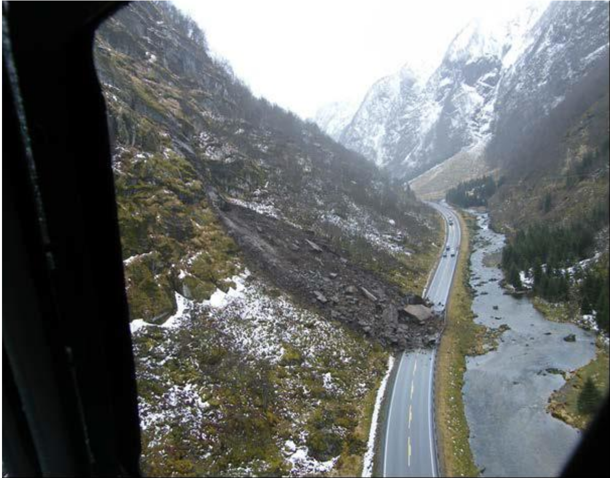
Photo: Landslide closing the E39 Highway at Insteffjorden in Sogn og Fjordane county, March 2010 (20090302, Njål Farestveit – NPRA)
