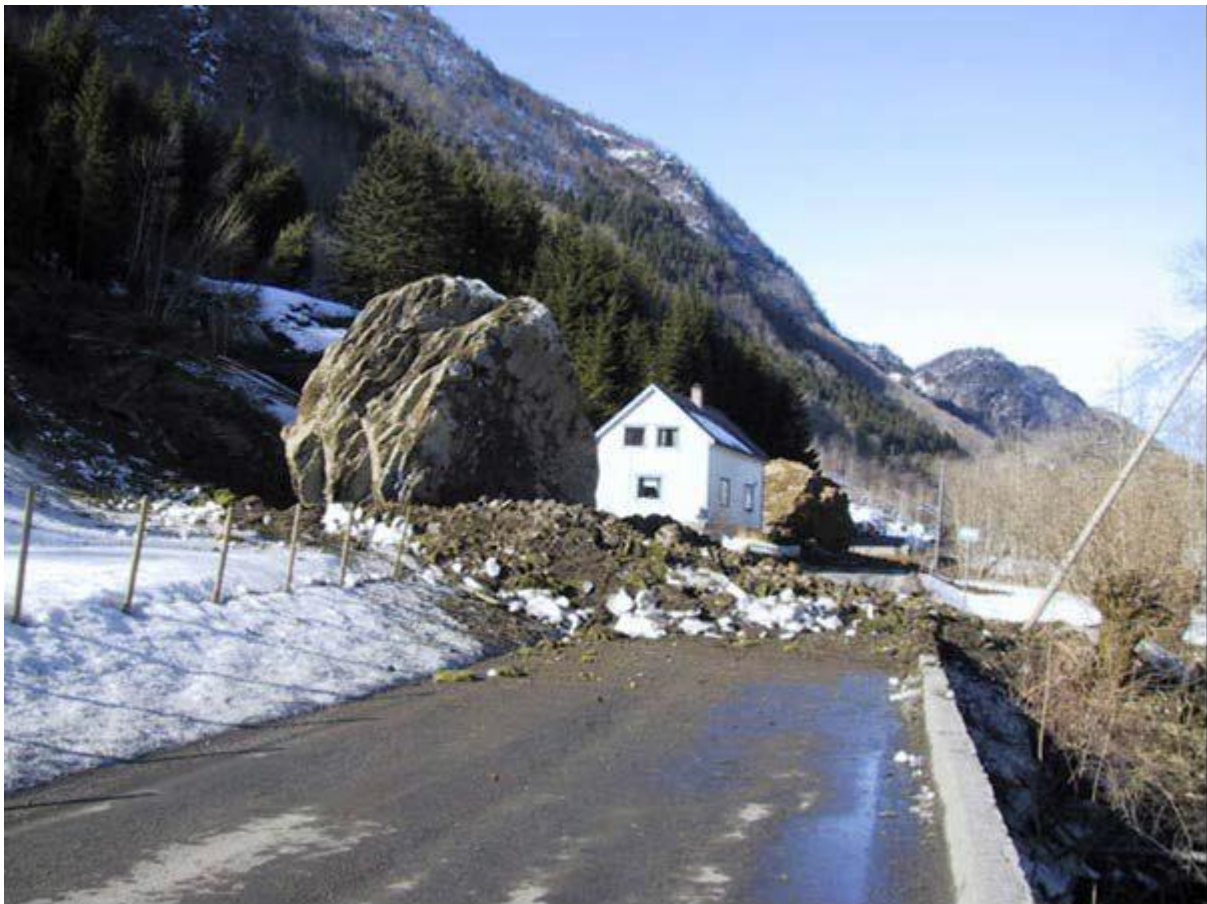
Photo: Rockfall by National Highway 48 Mundheim – Eikelandsosen in the county of Hordaland (20040309, Kvam local authority)
