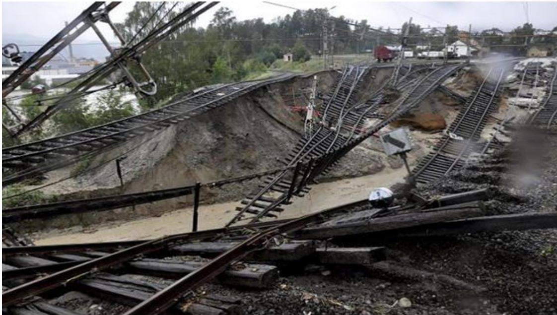
Photo: Notodden Railway Station in Telemark (20120723, NVE)
