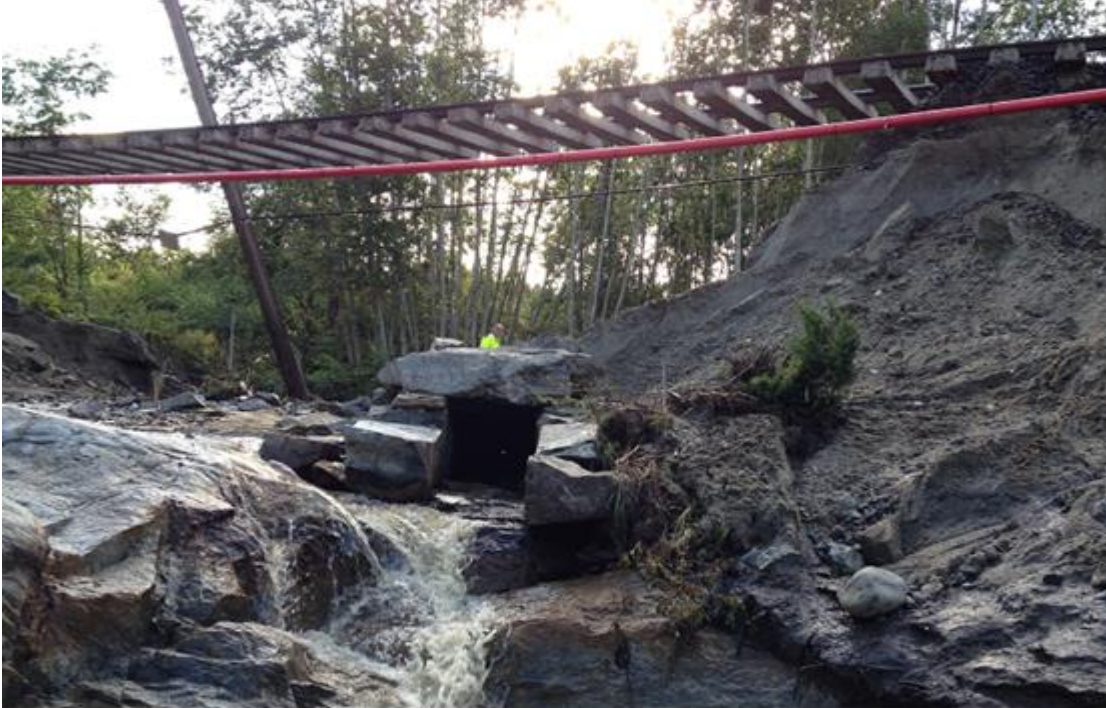
Photo: Surface runoff - the Randsfjord Line (20120807, Steinar Myrabø, JBV)
