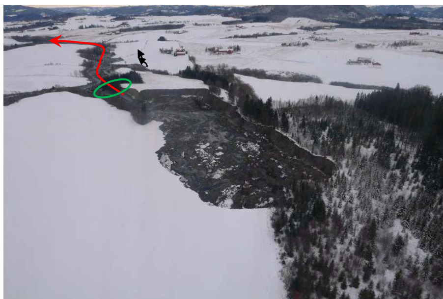
Figure 8. Bird's eye view of the 2012 Byneset quick-clay slide. The crater in the middle of the image is 8–10 m deep and about 350 m long. Probably it was erosion at the bend of the river that caused the initial failure (IF) that opened the narrow gate through which the main mass of the slide evacuated, following the course of the brook Brenselbekk (indicated by arrow). From (Lyche, 2012).
