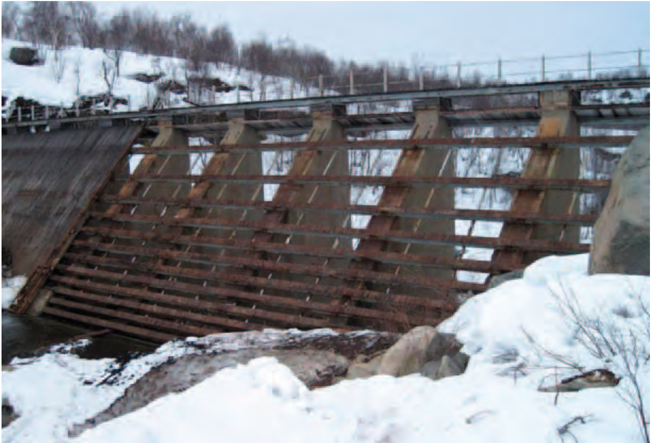
Dam under rehabilitering
