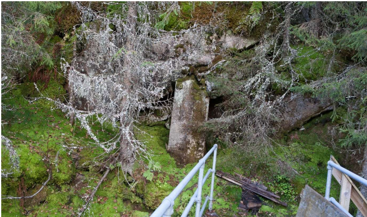
Betongfylling i fjellet (Stig Storheil/NVE 2016)
