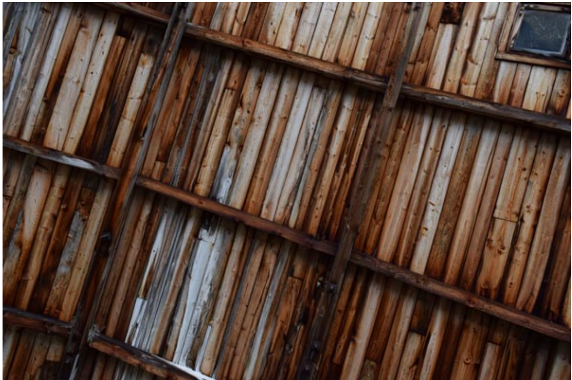
Fig 1. Navatn 03. Façade E wooden construction pattern.
