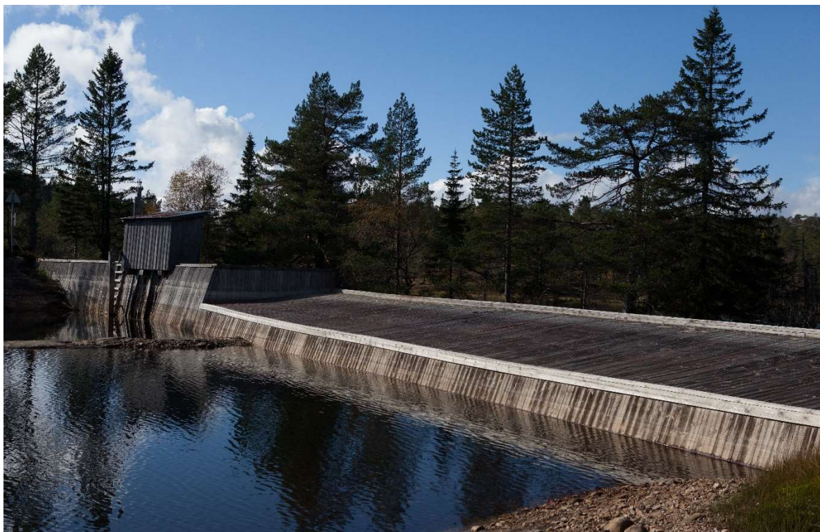
Langeraksvatn dam (Stig Storheil NVE 2016)
