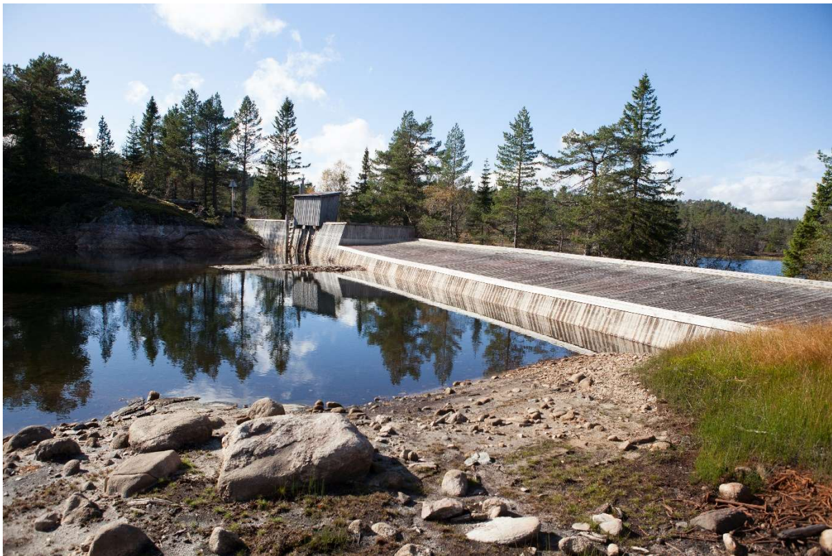
Langeraksvatn dam (Stig Storheil NVE 2016)
